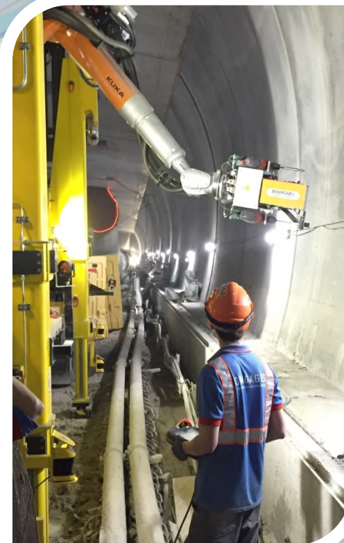
"ROBY 850" Concrete anchors installation robot
