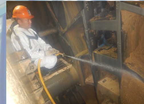
Worker cleaning cutterhead in pressurized excavation chamber
